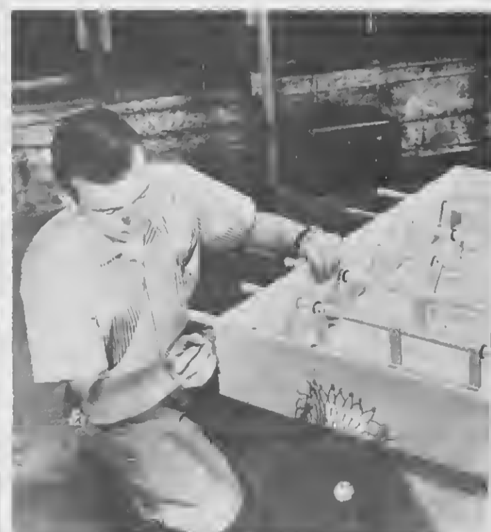
AFTER DOWELS have been inserted in holes, the final side of the box is positioned and either nailed or screwed together. Fish net or some similar material can be used for the net. DESPUES CU baranan worde pasá den e buraconan, e banda final di e caha ta worde poni na posicion y sea clabá of geschroef na otro. Tarai of material similar por worde usá pa e net.
